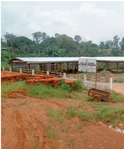
City centre ATOM just after its construction
