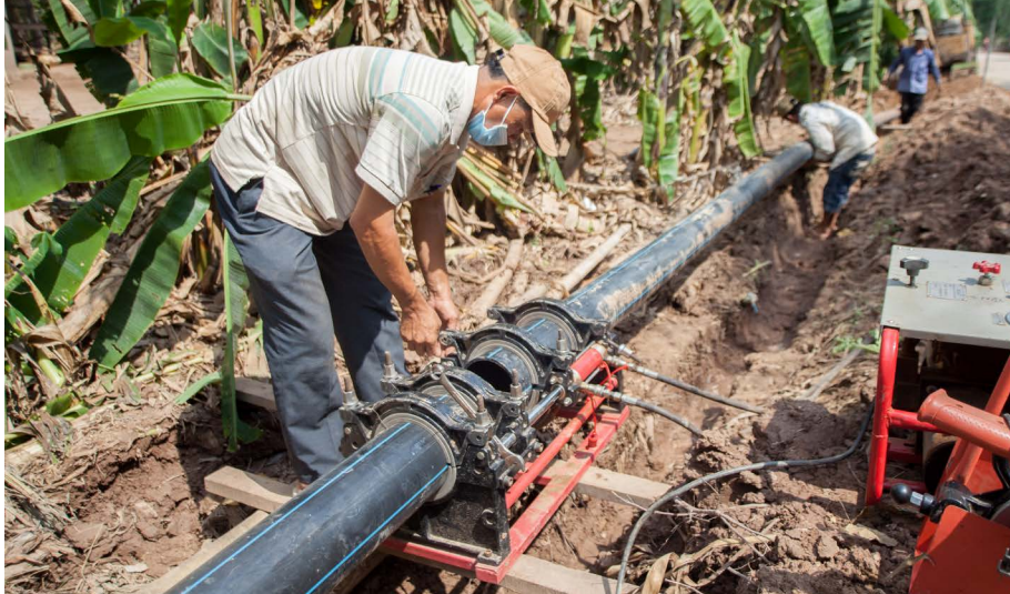
Water supply workers installing pipes extension © Germain Priour
