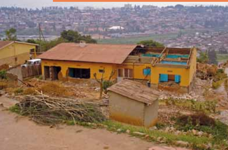
Unfinished building in Kiyovou neighbourhood in Kigali, Rwanda © Benjamin Michelon
